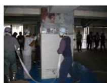
Retrofitting by polyester fiber sheet
