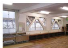
Retrofitted by V shaped steel brace
