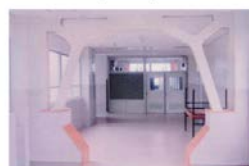
Retrofitted by Mansard shaped steel brace
