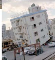
1 st floor collapse of a RC building
