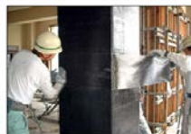
Retrofitting by carbon fiber sheet
