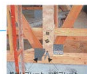
Brace end & Column base metal joint retrofitting
