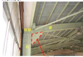
Retrofitting by Rib plate
