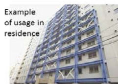
Retrofitted with brace
