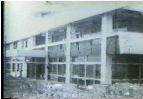
1964 Niigata Earthquake: Sinking terminal building
